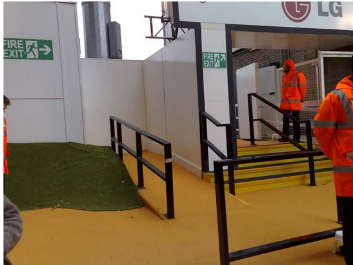
Figure 7: Disabled away supporters' area, new platform and ramp.
